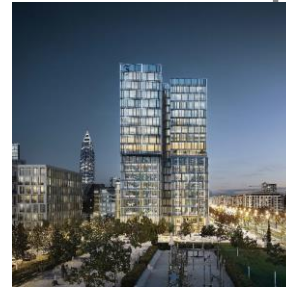
FAZ Tower, Frankfurt
