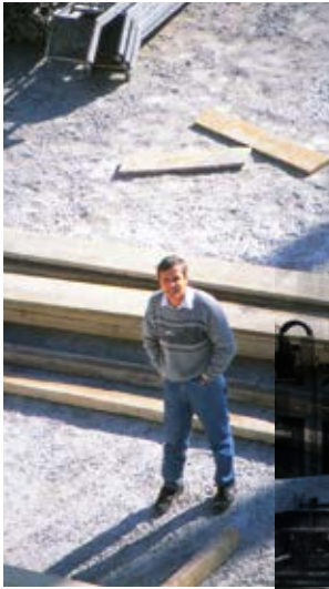
1989. Hermann Blumer during construction of the Lignatur AG workshop
