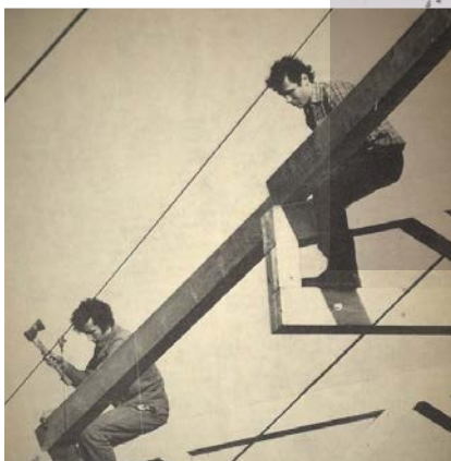
1974. Hermann Blumer (top right) during construction of the Stüdl Hall in the Swiss town of Herisau
