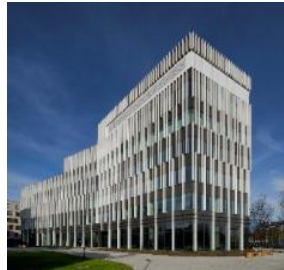
Kotlarska 11 Krakow GLA: 11,000 m 2 Completion: 2017
