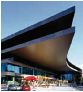
Neue Mitte Lehen Office and Retail, Salzburg
