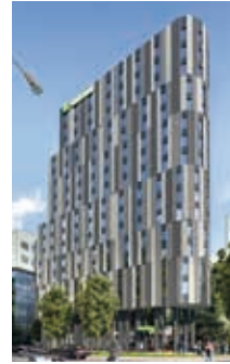
Holiday Inn Warsaw City Centre Hotel, Warsaw
