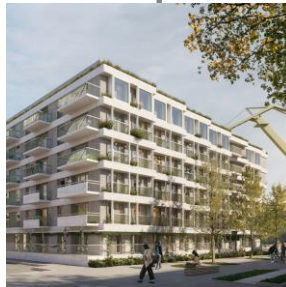
Timber View, Mainz Apartments: 176 Completion: Q4/26
