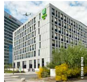
Airport hotel Gateway Gardens, Frankfurt Rooms: 288
