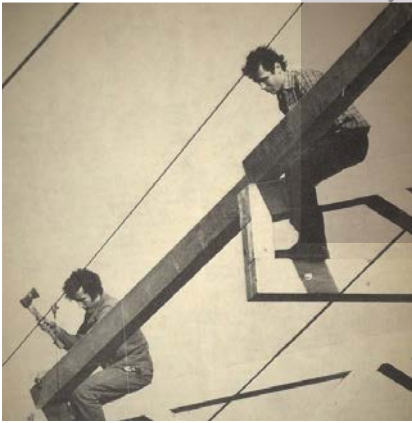
1974. Hermann Blumer (top right) during construction of the Stüdl Hall in the Swiss town of Herisau
