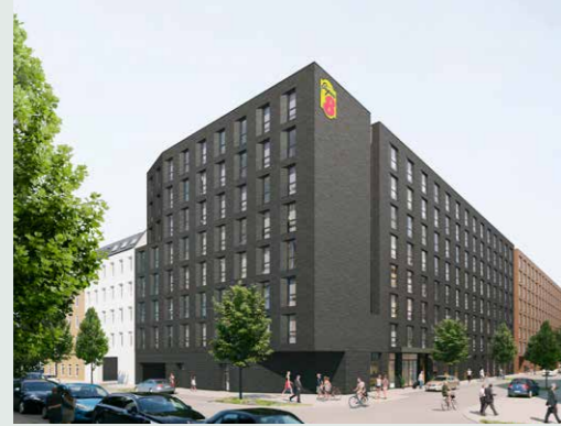
Holiday Inn & Super 8 Eiffestraße Hamburg Rooms: 592 Completion: 2019
