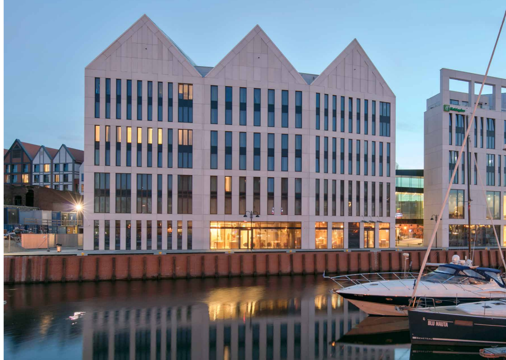
On the water, in "Flow": The Holiday Inn Gdansk City Centre
