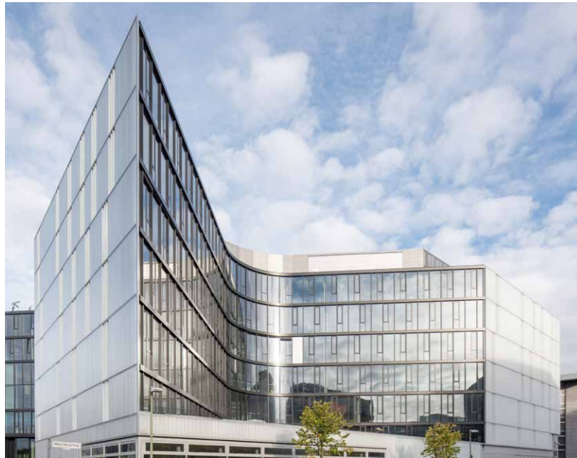
In tune with growth: The Zalando headquarters, Berlin
